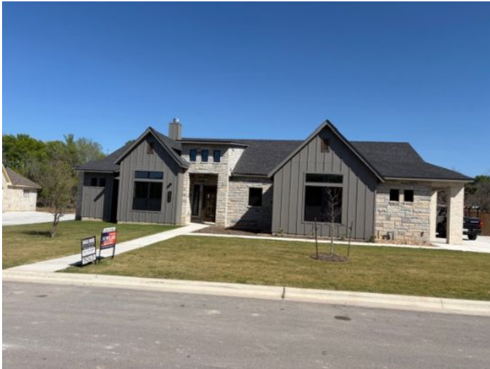
Exterior Walls - Brick Veneer, Stone Veneer, Board and Batten Siding
