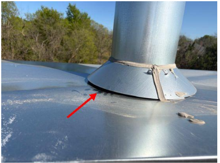
Gap between Storm Collar and Chase Cover
