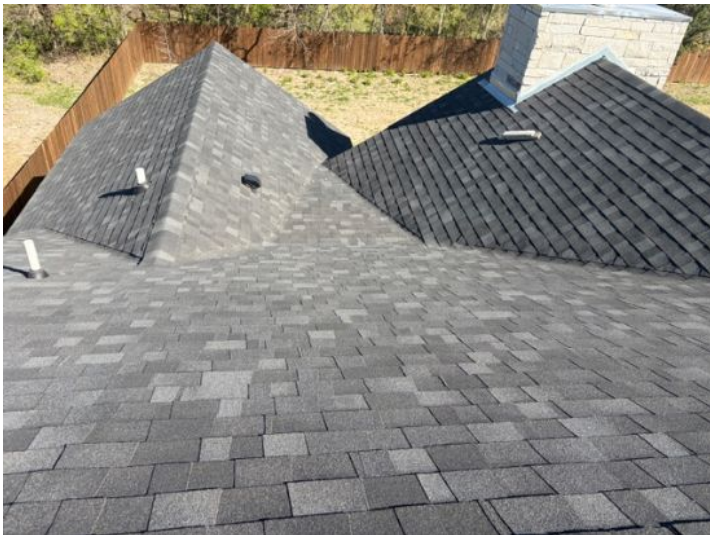
Roof Covering Material - Architectural Asphalt Shingles
