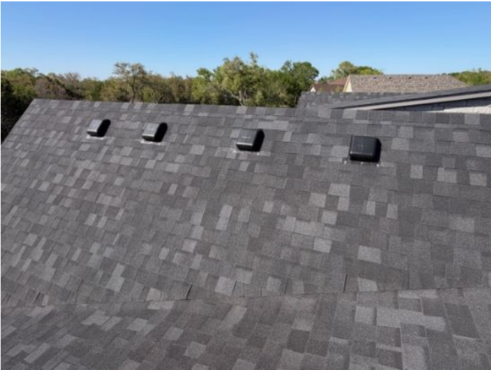
Unconditioned Attic Space (Above Garage) Vents
