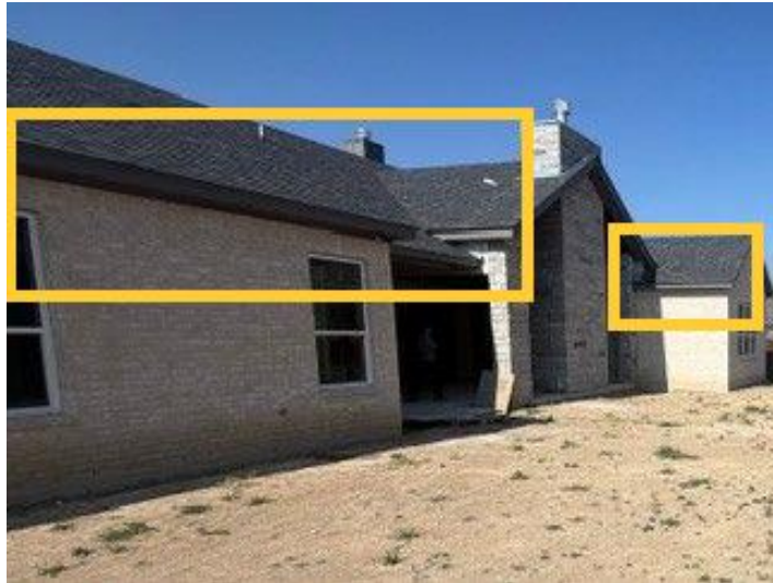
Gutter System Recommended
