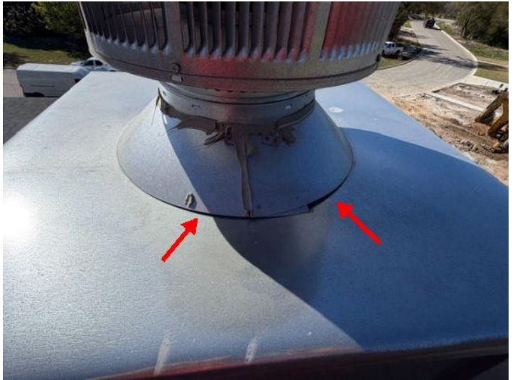
Gap between Storm Collar and Chase Cover
