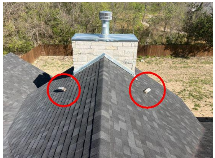
2x4s Nailed to the Roof
