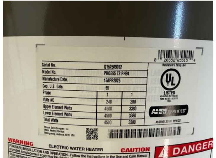
Traditional Tank Water Heater Data Plate
