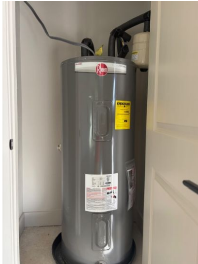
Traditional Tank Water Heater
