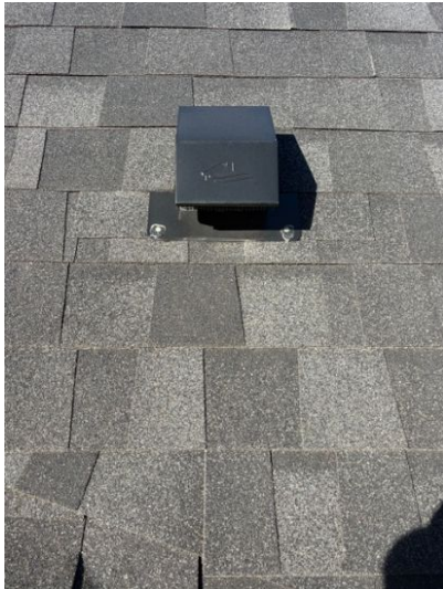
Bath Fan/Exhaust Fan Vent
