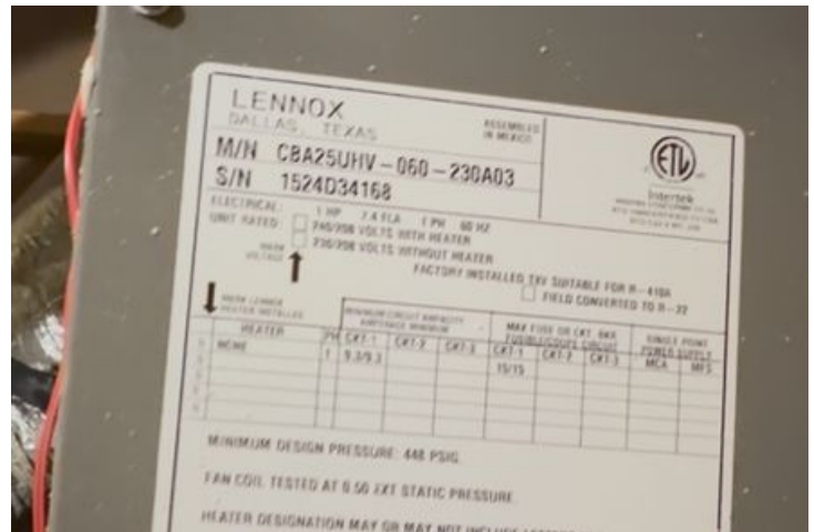
HVAC Furnace Data Plate
